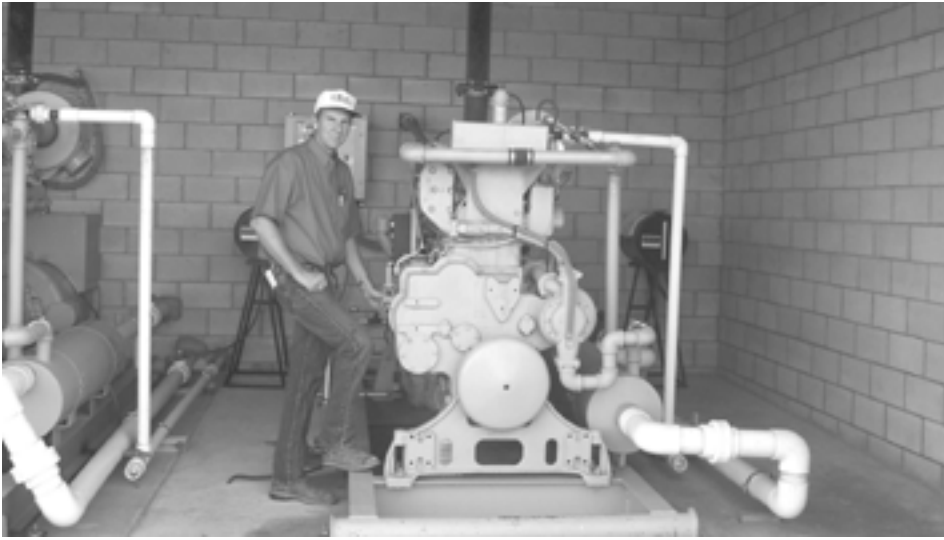
Lindsay dairyman Rob Hilardes has installed a methane digester system to produce electricity from dairy waste. Photo courtesy of Western United Dairywomen
